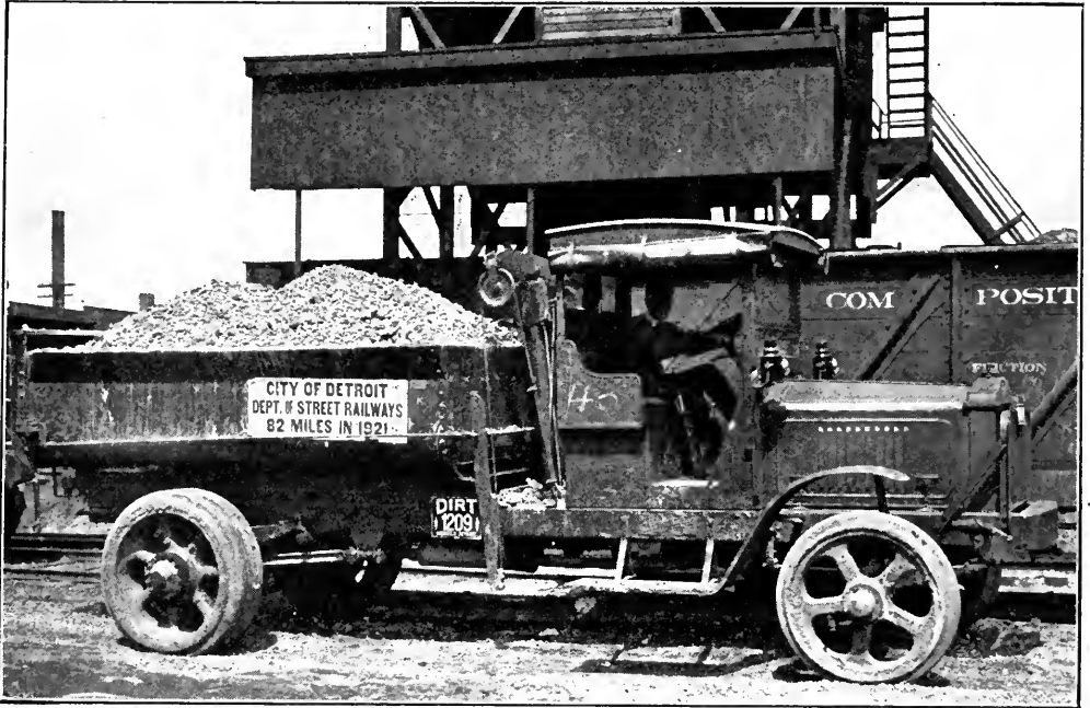
A STANDARD TRUCK USED FOR HAULING BALLAST BY THE DEPARTMENT OF STREET RAILWAYS, DETROIT, MICH.
